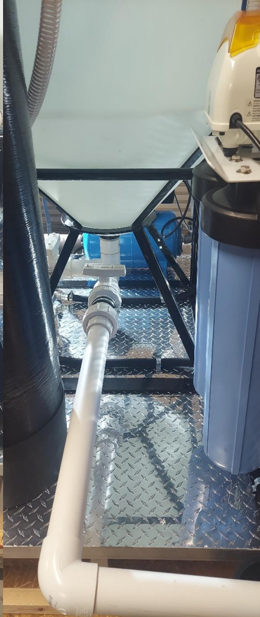
To circulate the Holding Tank water back onto the Wash Pad
